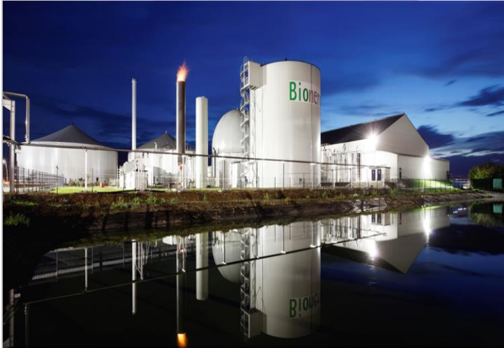
ORGANICS2POWER BIOGAS BIODIESEL
